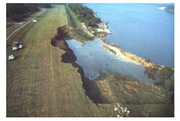
Picture of levee breach
